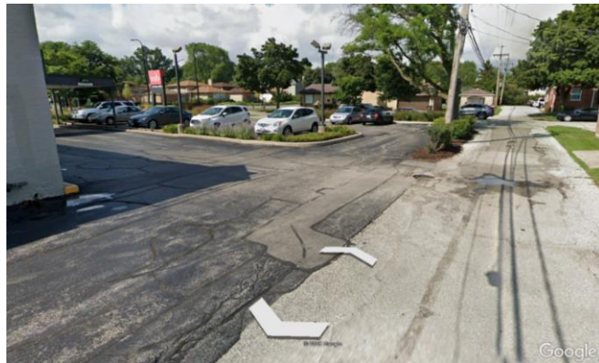
Existing Condition between the Subject Property and Alley to the North
